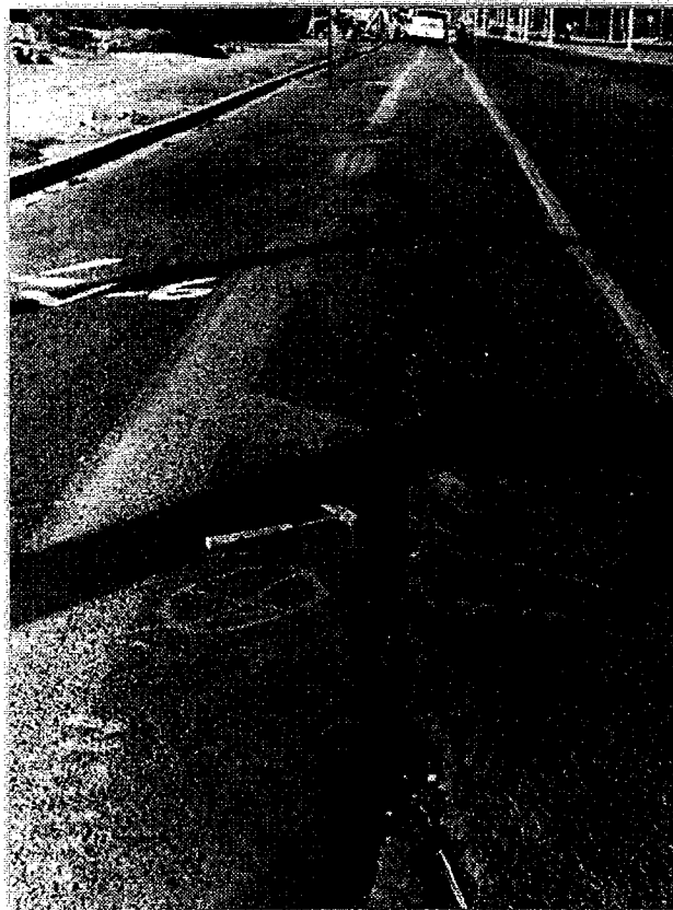
Figure 3a: Sulfate heave distress on Stewart Avenue in Las Vegas, NV (Hunter, 1988).
